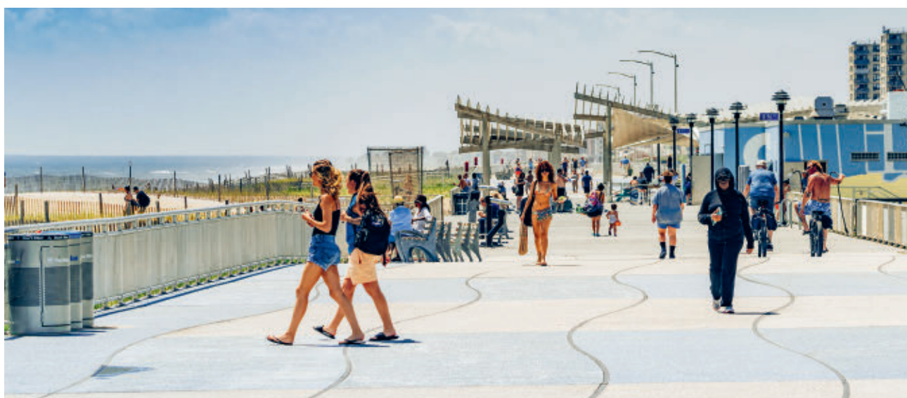
Skanska has rebuilt the Rockaway Beach Boardwalk, in New York, USA, which was destroyed in the hurricane Sandy 2012. The new boardwalk is elevated and has a steel-reinforced concrete deck.
