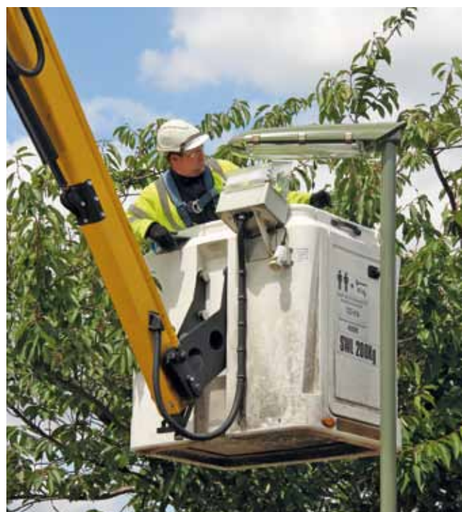
The newly installed street lighting network in Surrey, U.K. is energy-efficient thanks to a central control system.
