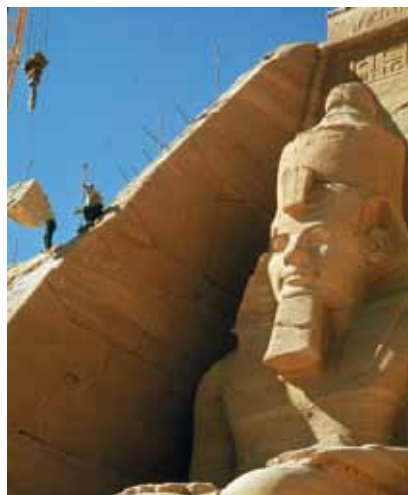
1963 Abu Simbel was saved from being submerged behind a new dam on the Nile in Egypt. The 3,000-year-old temple was sawn into cubes and lifted 60 meters (200 ft.) higher.
