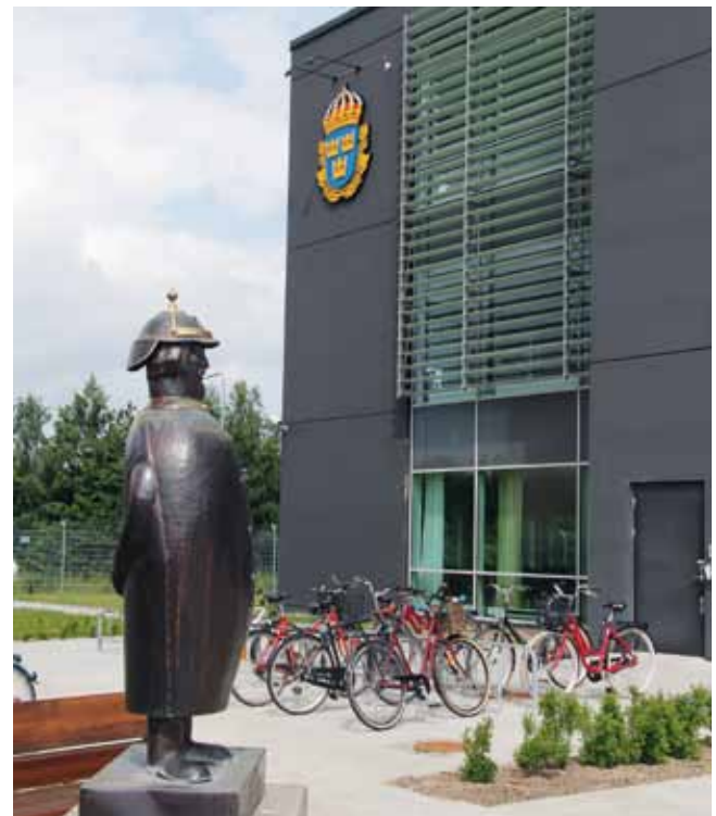
One of two police buildings that Skanska has been constructing in Malmö, Sweden.
