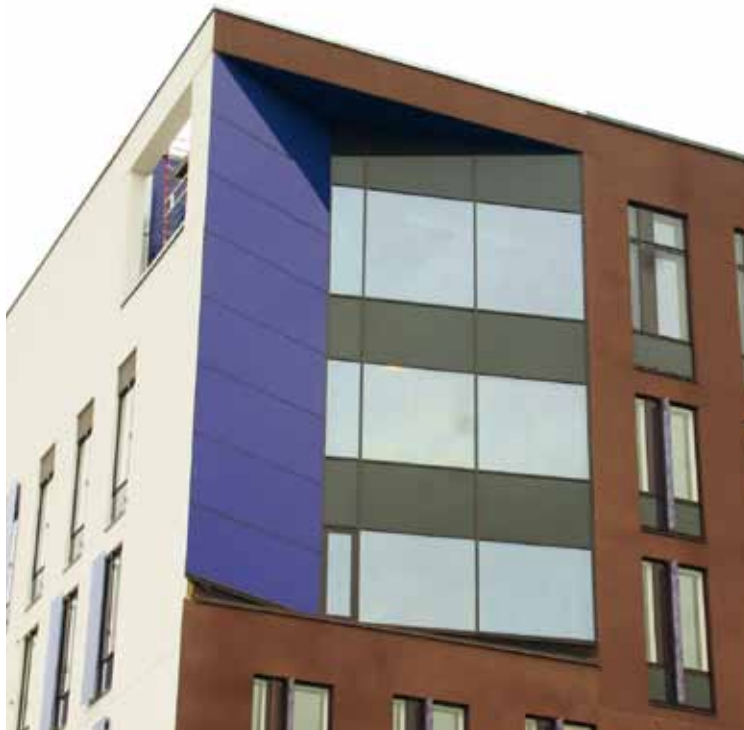
Skanska's new Ruskasuo office building in Helsinki, Finland.
