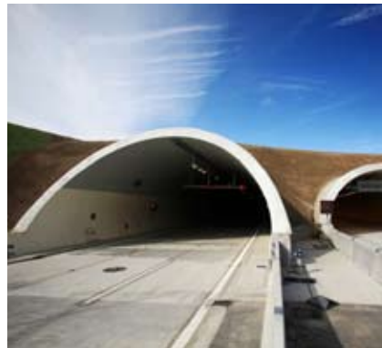
Two tunnels that are 2 km (1.2 mi.) long are part of the ring road around Prague, Czech Republic.
