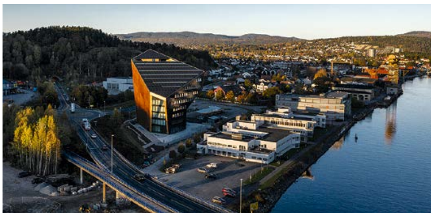
Powerhouse Telemark located in Porsgrunn, Norway, are one of the most energy efficient and environmentally-friendly buildings in the world.
