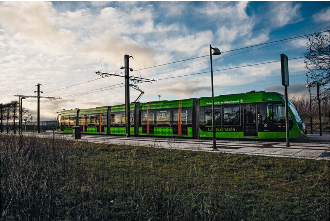
The new tramline Skanska built is connecting the ESS in Lund, Sweden with the central parts of Lund.
